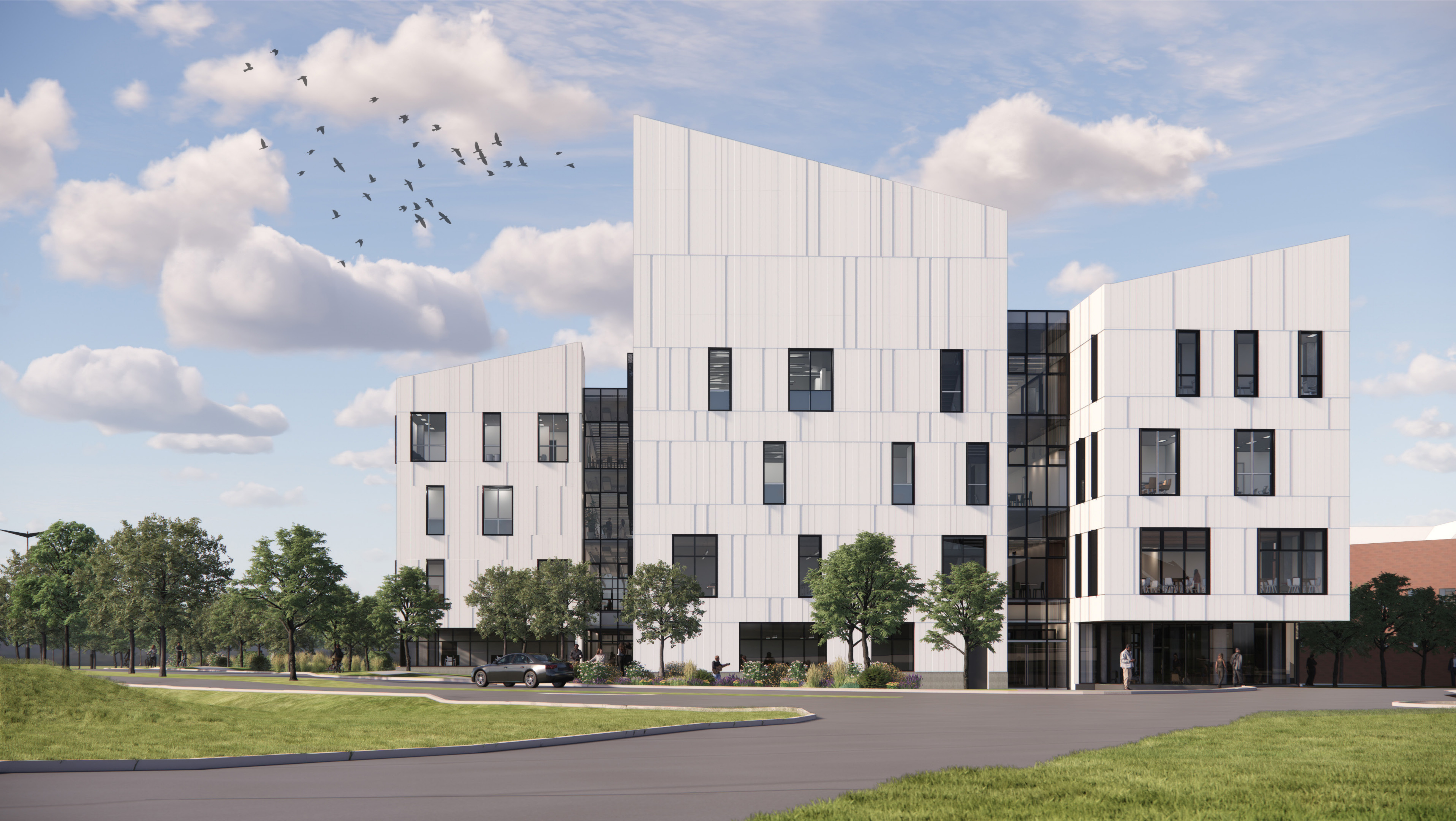
EXTERIOR VIEW FROM SOUTH
